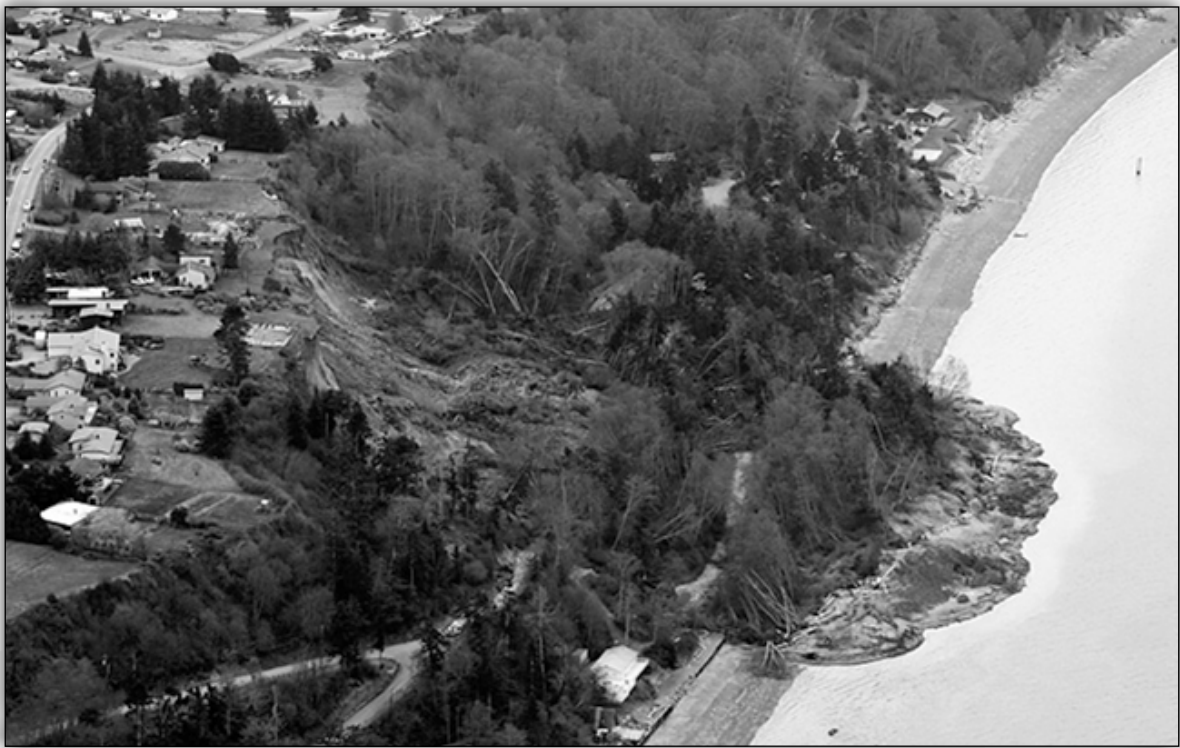
Landslide near Bush Point, Whidbey Island. (#521)
